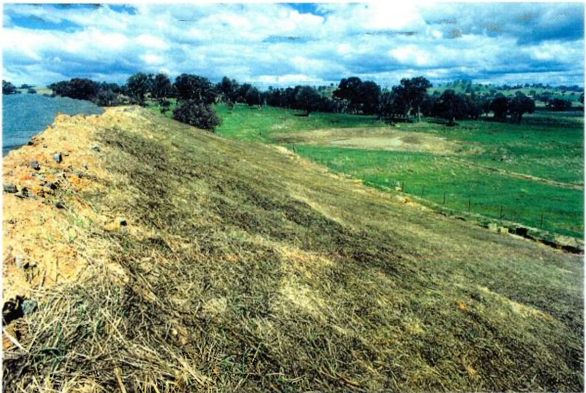
Photo No.2 Western flank of the existing section of Stockpile Area No.2 showing the 1V:3H batter and recent grass seeding.
